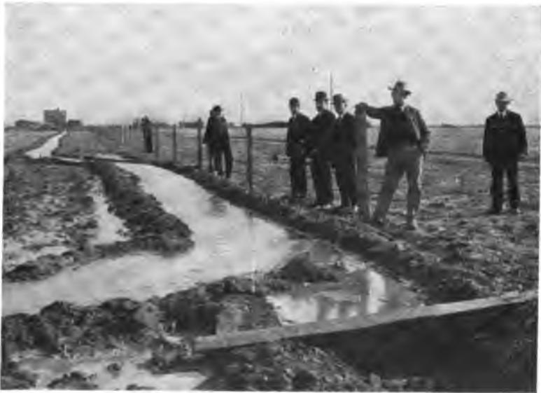
FIG. 33.—Diverting Water from Head Ditch by Canvas Dam, Shoshone Valley, Wyoming.
